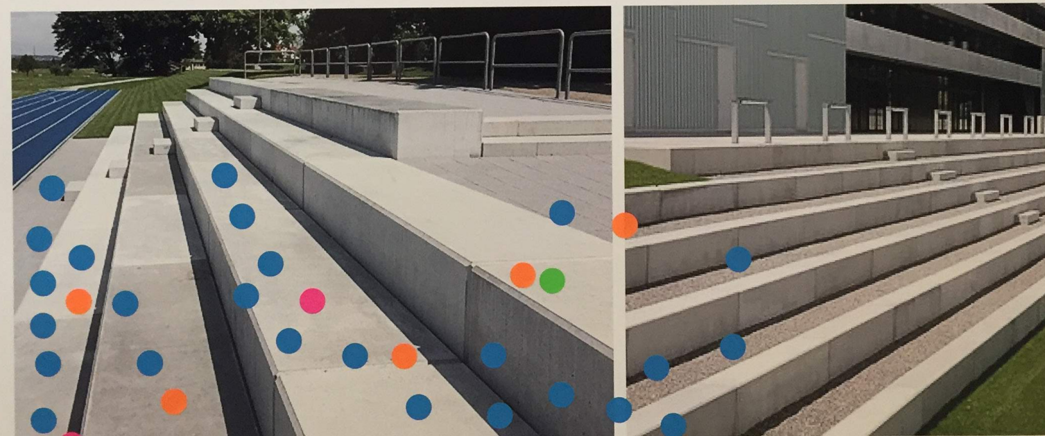
Integrated, concrete platform seating along slope
